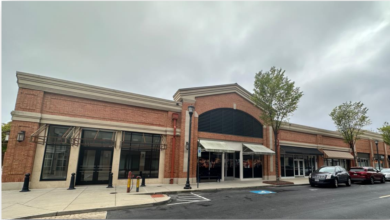
Existing Bldg D Vacant Retail Space (Unoccupied for 5 Years*)
