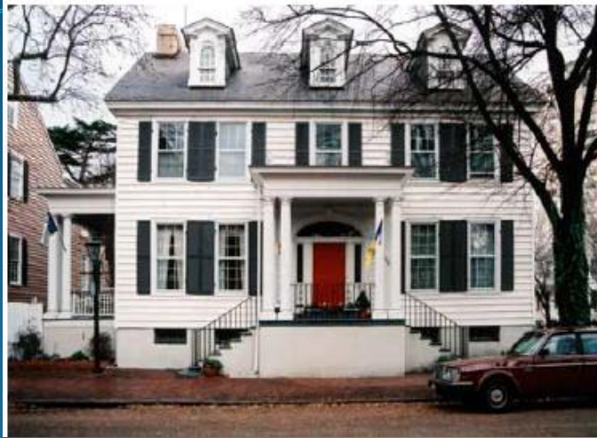
Buckroe Colonial Revival
