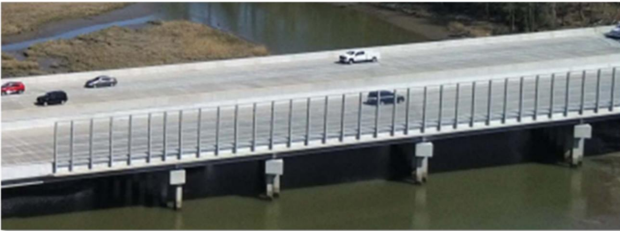
Transparent Structure-Mounted Noise Barriers (Hampton River Bridges)
