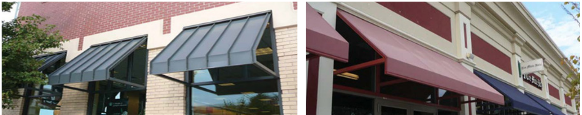
Figure 5: Awnings and canopies are covers or partial roofs that extend over building entrances or other openings in order to shield pedestrians from the weather. Awnings and canopies shall be designed to project over individual entrances and openings, rather than extending the length of the building face.
