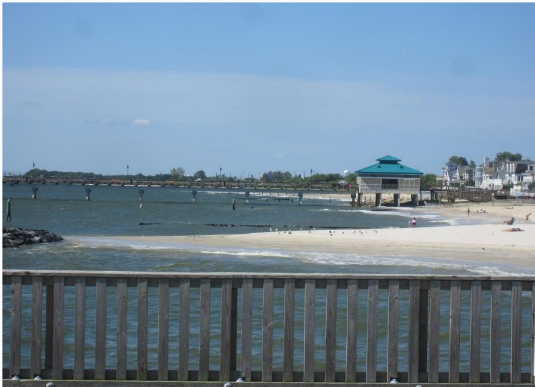
Offshore Rock Breakwater
