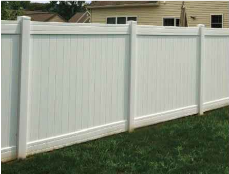
6' HEIGHT WHITE VINYL/PVC PRIVACY FENCE WITH 5" X 5" POSTS, SET IN CONCRETE AT 8' O.C.. INSTALL PER MANUFACTURERS SPECIFICATION AND RECOMMENDATION.
