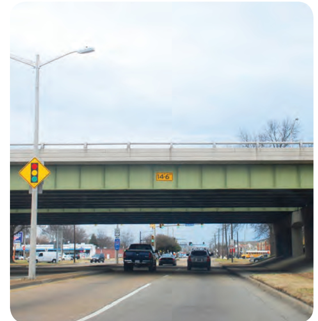
Constrained conditions under overpass at Mercury Boulevard limit opportunities for retrofitting the roadway with bicycle and pedestrian facilities. (Source: Rhodeside & Harwell)
