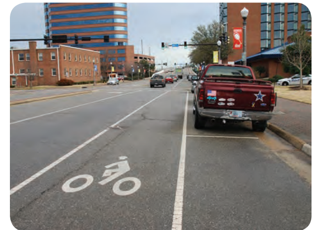
Figure 2: Examples of Hampton's Existing Facilities
