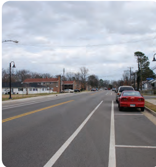
Figure 40: Existing Conditions in Buckroe Bike lanes on Pembroke Avenue lack some markings. (Source: Rhodeside & Harwell)
