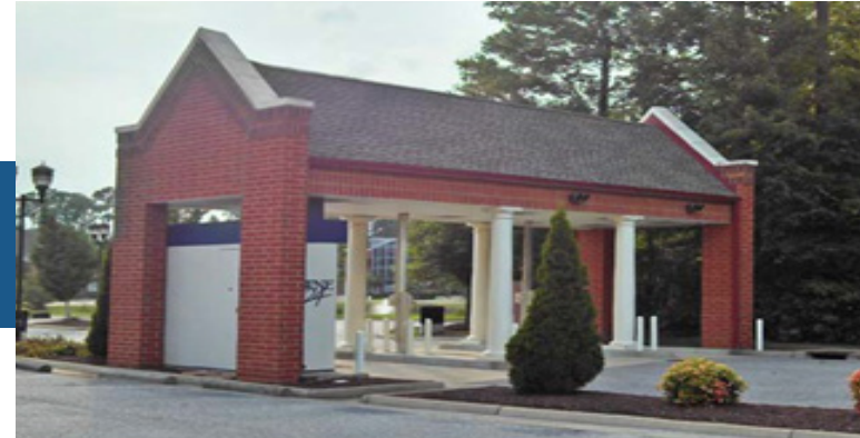
Figure 9: Attached and detached drive-through coverings that incorporate the building design and include building materials and sloped roofs that mimic the primary structure.
