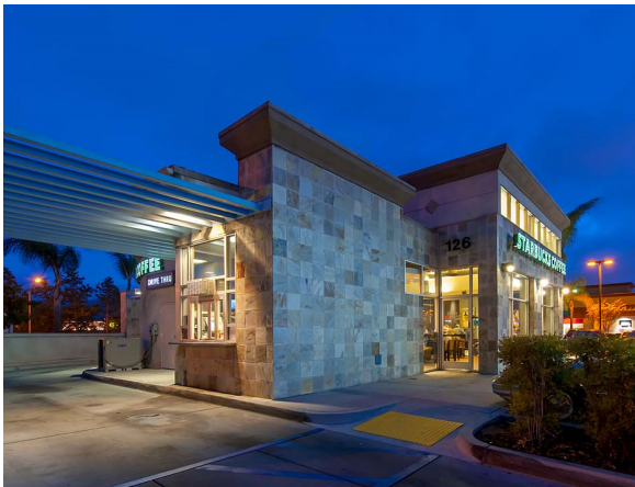
Figure 9: Attached and detached drive-through coverings that incorporate the building design and include building materials and sloped roofs that mimic the primary structure.
