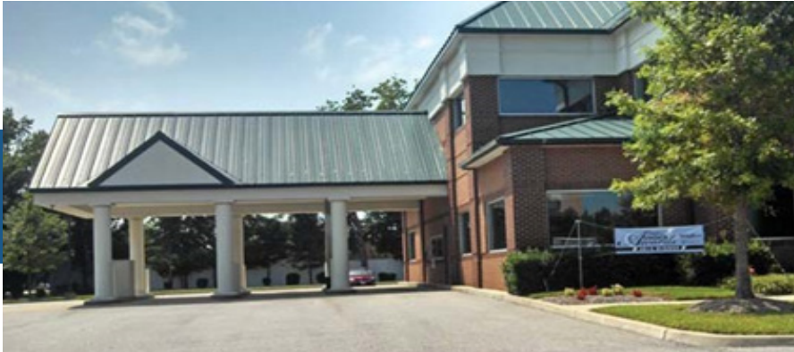
Figure 9: Attached and detached drive-through coverings that incorporate the building design and include building materials and sloped roofs that mimic the primary structure.
