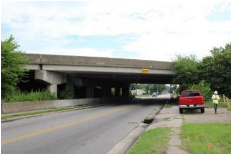
I-64 over Riprap Road
