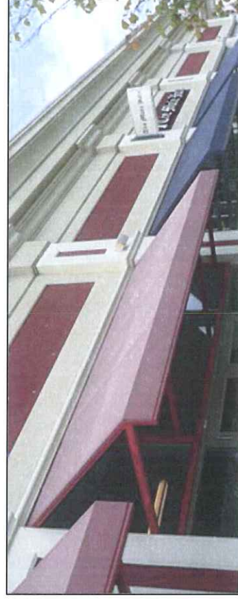
Figure 6: Awnings and canopies are covers or partial roofs that extend over building entrances or other openings in order to shield pedestrians from the weather. Awnings and canopies shall be designed to project over individual entrances and openings, rather than extending the length of the building face.
