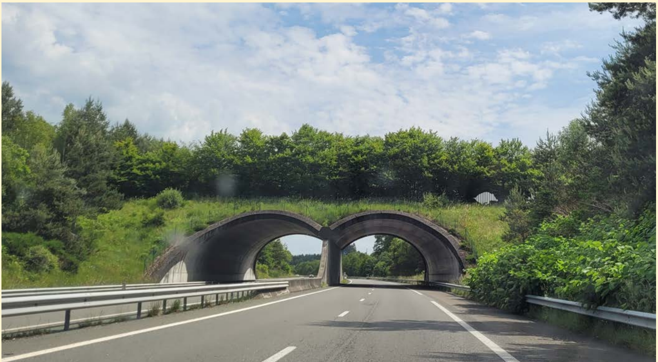
Wildlife bridges can be used in rural areas for large mammals to cross roads without conflicts. In cities, smaller mammals and amphibians can benefit from wildlife tunnels under roads.
