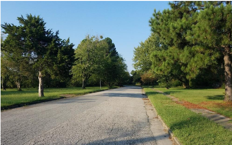
Freeman Drive Relocation
