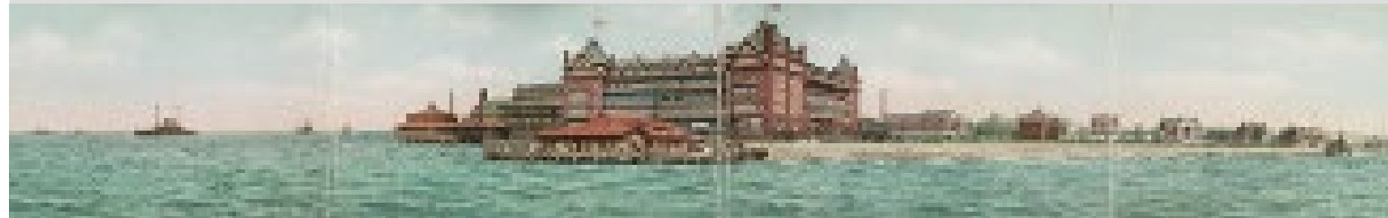
(above) The postcard depicts the original Chamberlin hotel built in 1894 and destroyed by fire in 1920. Built in 1927 and 1928, the existing Chamberlin building was designed by Whitney Warren. Source: Library of Congress
