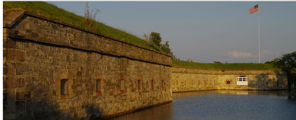
(above) Fort Monroe, known as "Freedom's Fortress", is the largest stone fort in the United States and was constructed between 1819 and 1834. Source: NPS Photo
