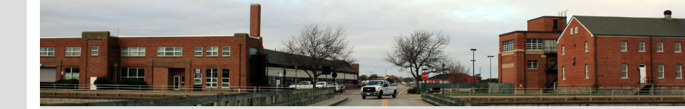
(right) From the North Gate of the Inner Fort, this view of the North Gate area shows many large structures with potential for reuse in Fort Monroe's employment focus area.
