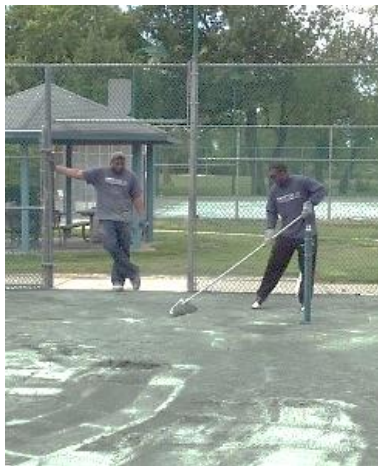
Woodland Tennis Court Resurfacing
