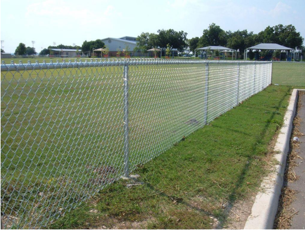
Figure 2: Galvanized Chain Link Fence
