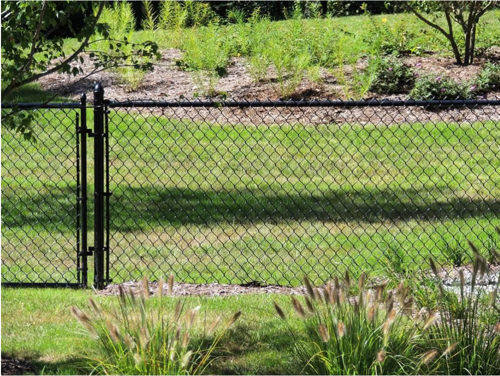
Figure 3: Vinyl Coated Chain Link Fence
