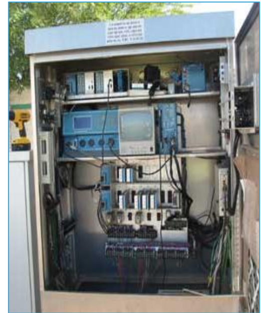
Completed 64 fiber optic repairs
