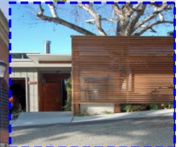
WOOD SLAT SCREEN DETAIL
