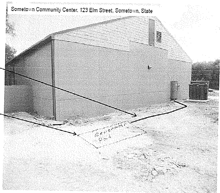
Figure 4. Ground-level photograph showing proposed ground disturbance area.
