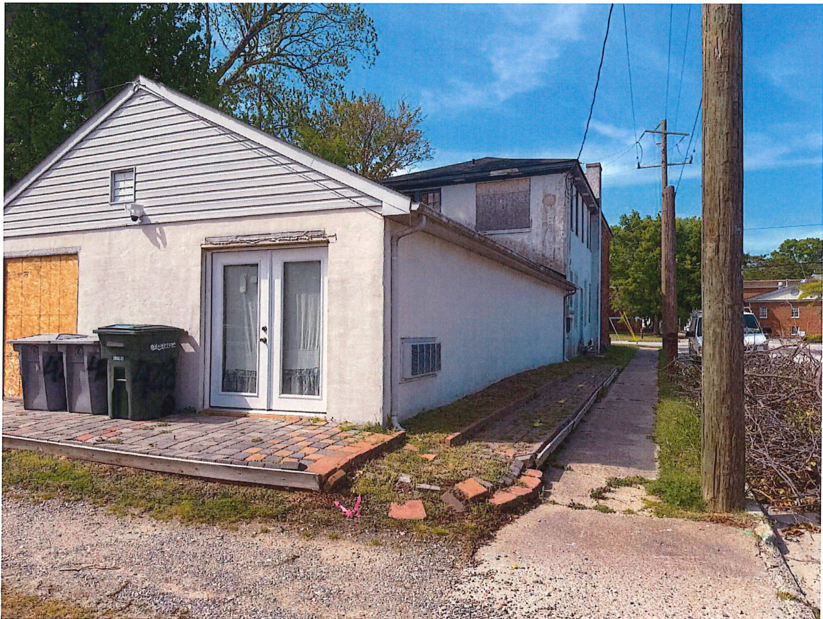
Figure 1: Side Yard adjacent to Sidewalk showing Building located on 4218 Victoria Blvd
