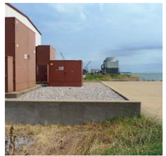
Above: Utility equipment that has recently been elevated on concrete pads.
