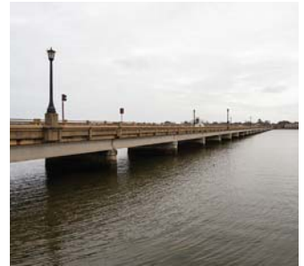
Above: The N. King St. bridge is a vulnerable structure because of its low elevation, and also has utility systems directly attached that have frozen before.
