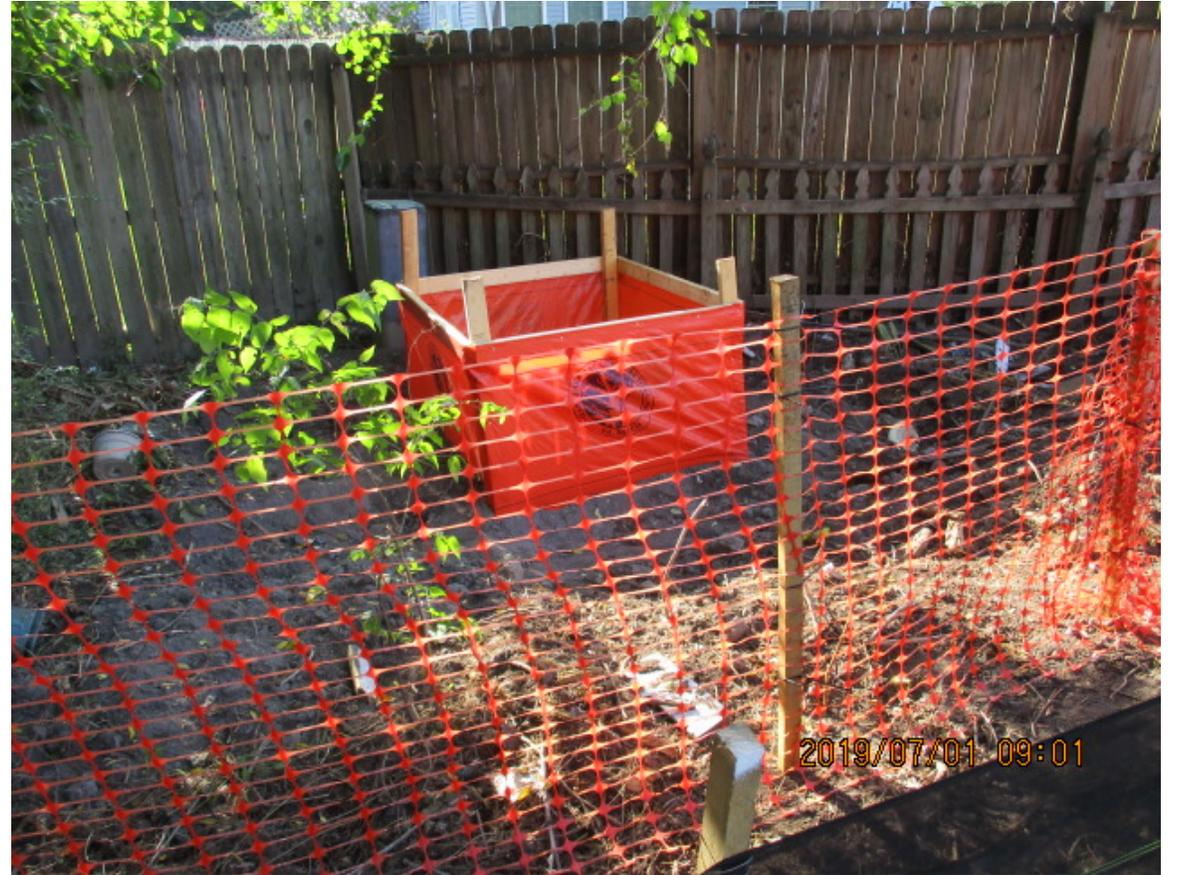
E&S inspections such as the silt fence protecting the Hampton River during roadway improvements and boxed inlet protection during subdivision construction
