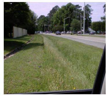
High grass to filter stormwater runoff in ditches is an exemption
